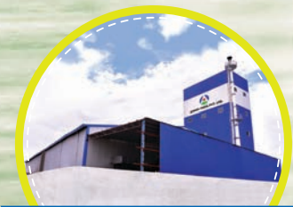
NEW PLANT AT PANCHLA, WEST BENGAL
