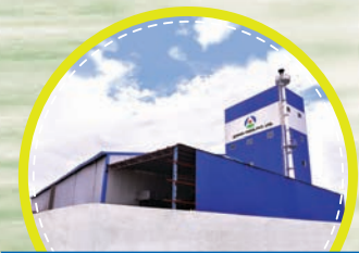
NEW PLANT AT PANCHLA, WEST BENGAL
