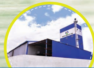
NEW PLANT AT PANCHLA, WEST BENGAL
