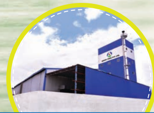
NEW PLANT AT PANCHLA, WEST BENGAL
