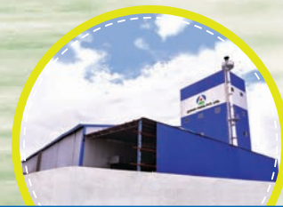
NEW PLANT AT PANCHLA, WEST BENGAL
