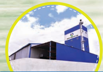
NEW PLANT AT PANCHLA, WEST BENGAL
