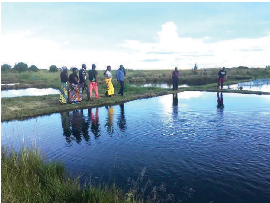
Fish ponds with very low dykes, such as these in Zambia, are vulnerable to flooding.
