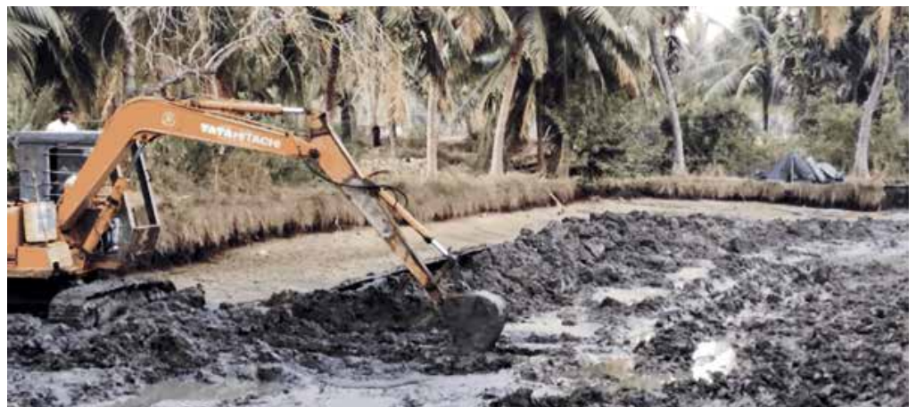
The SSFI team uses an excavator for sludge removal at a shrimp pond
